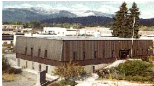
Boundary County District Library, Bonners Ferry, Idaho.
